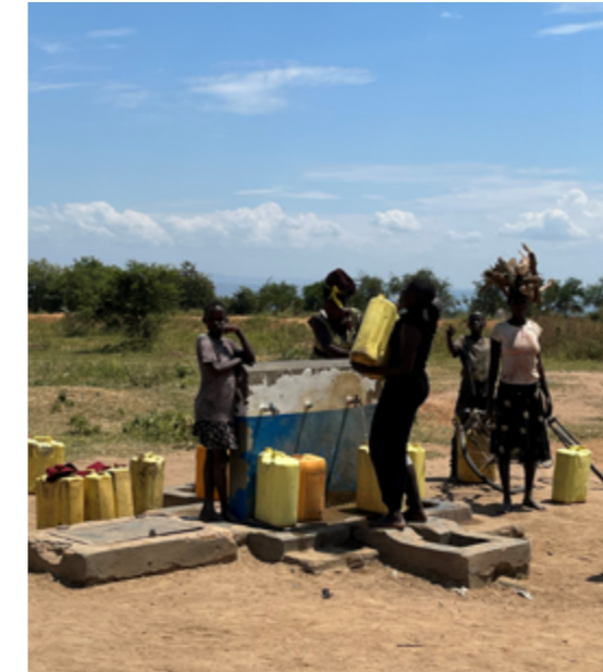
Kirama water project.
